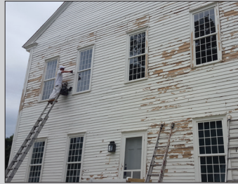
The Jaffrey Meetinghouse (1775) getting a fresh coat of paint on the east gable end. We also did some painting on the Tower and the ceiling inside.
